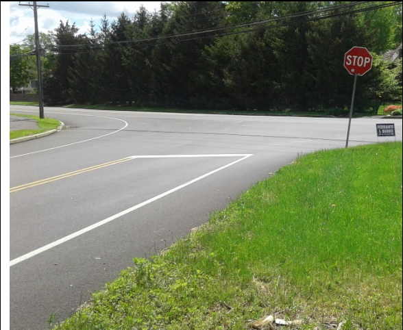
Dolington and Quarry intersection
