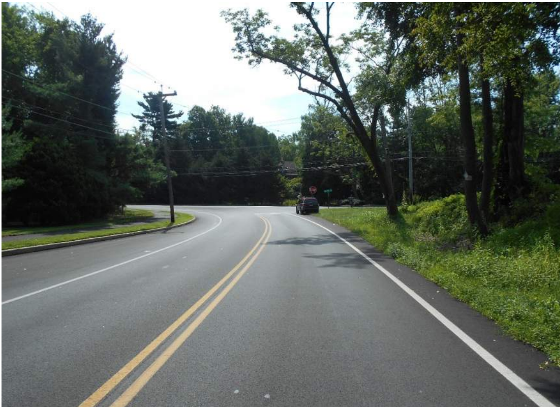
Direction / Road: SB Dolington Road Approach / Departure: Approach Distance: 200'
