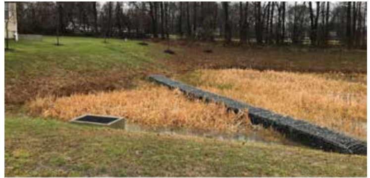
(Water Quality Basin at the Freeman's Farm Development on Big Oak Rd)
