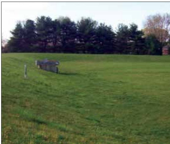
(Basin along Lindenhurst Rd.)
